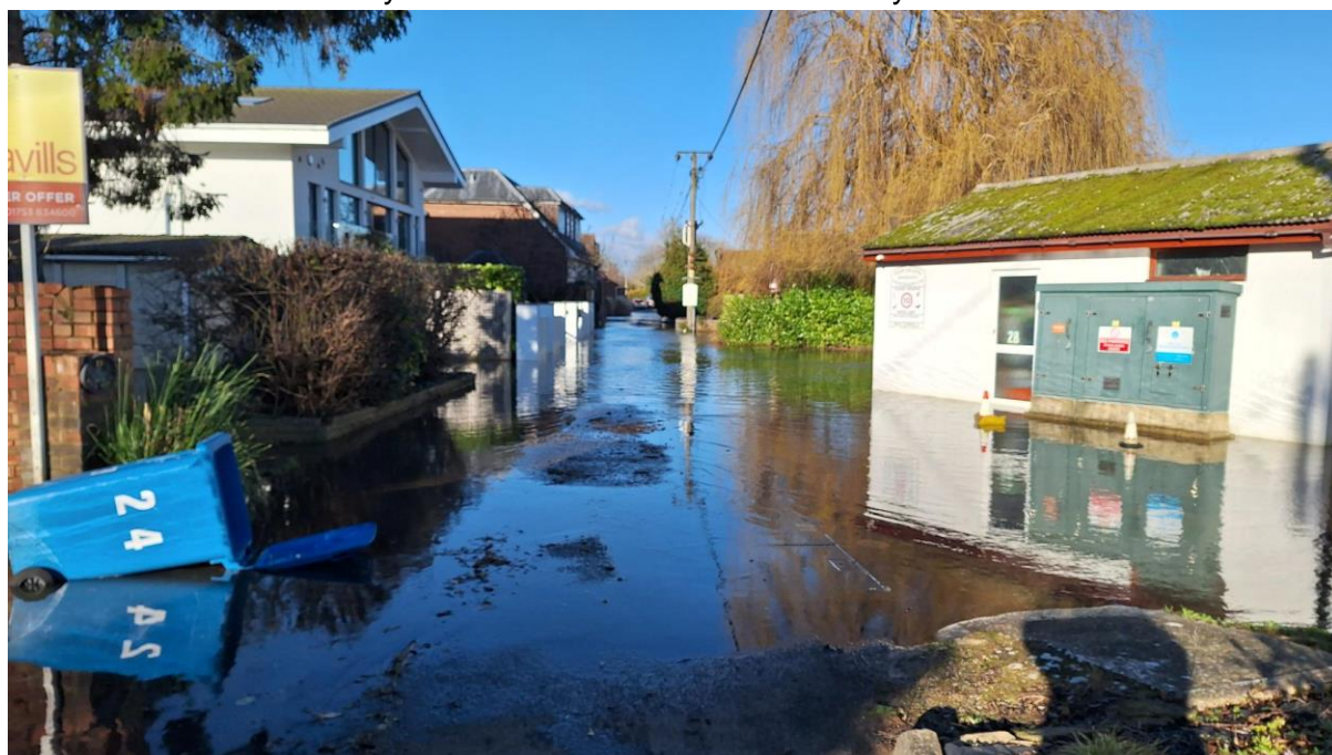
Figure 26- Photo showing flooding at Ham Island
