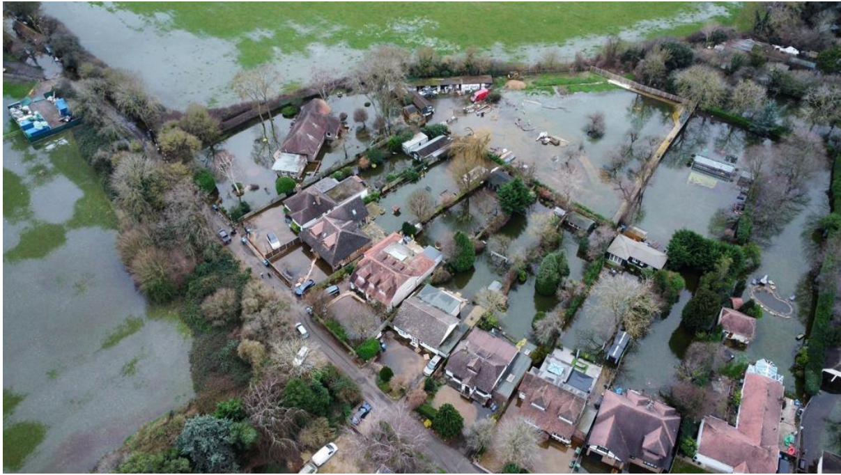
Figure 25-Photo showing flooding to properties around Garson Lane, Wraybury
